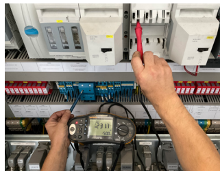
Loop impedance measurement
